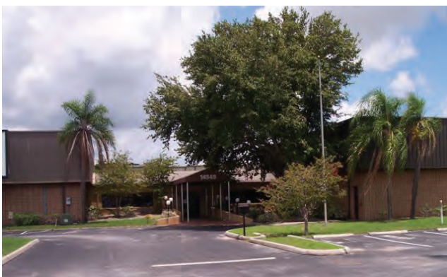
View of main entrance to front building
