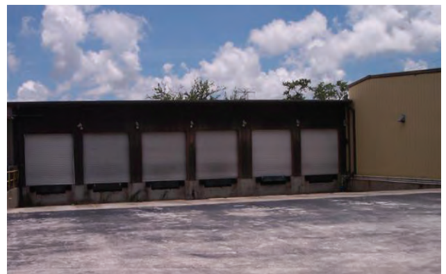
6 truck wells in back loading area
