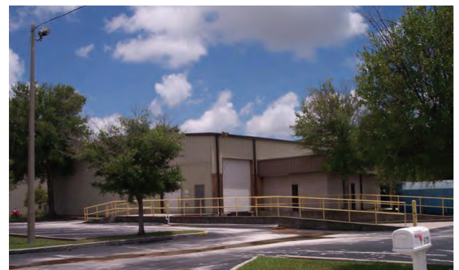
Truck well & loading dock on a back building
