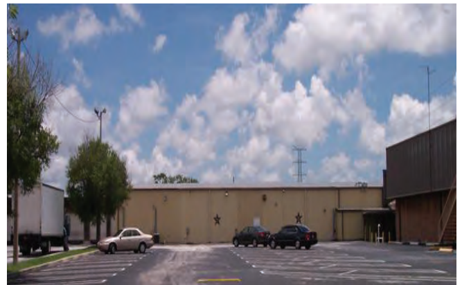
View of smaller connecting warehouse area
